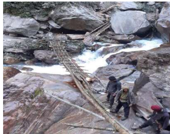
Figure 10: Up-gradation of foot trail and construction of temporary bridge ( fadke )
