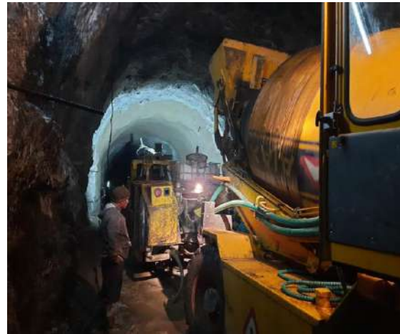
Figure 5: Shotcrete work inside road tunnel
